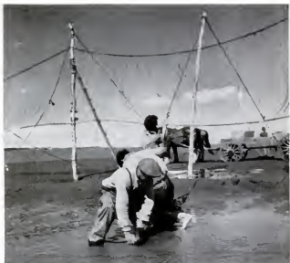
ATTACHING ROPES from poles to the guy stakes holds the net in place. Ninety of these sturdy birch poles are needed to hold up the 1,000-foot net.
